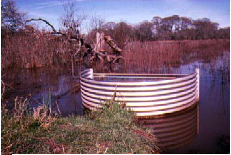
A flashboard riser box attaches to a pipe installed in a levee to create a shallow water wetland for wildlife.
